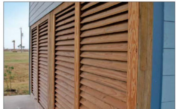
Figure 2-21. Louvers installed beneath an elevated house are a good alternative to breakaway walls SOURCE: FEMA P-499 2010
