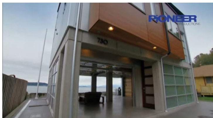
Overhead Bay Doors – Act as privacy screens when needed. They open up to allow for an outdoor lounge space, and be closed when not in use. After emailing the creator of these overhead bay doors, Architect Dan Nelson suggested I should alarm these doors for extra protection. If a storm is coming, these doors can be opened to allow flood waters to pass through with ease. I have also installed flood vents in my design incase the home owners are not home when a storm is coming.
